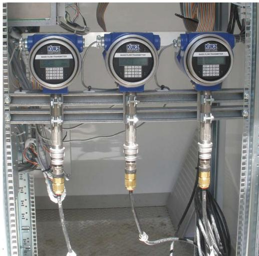
**Figure 2-26. Cable gland example with braided shielded cable**
