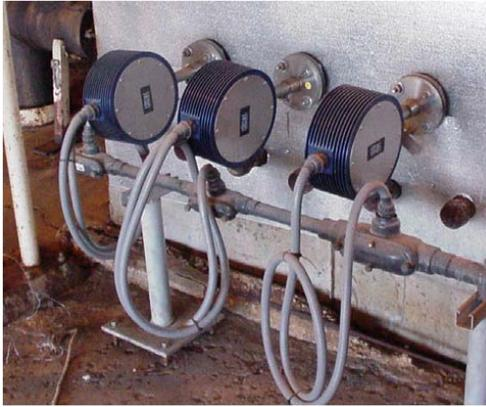
**Figure 2-24. Flex sensor connection for service loop, TA version using liquid tight conduit**
